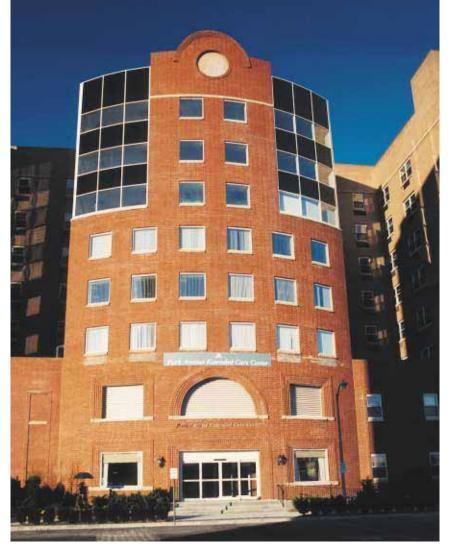
The Park Avenue Extended Care Center in Long Beach, N.Y., benefited from the use of bollowcore slabs, which facilitated sound control and offered fire resistance. The precast floor system also allowed 34-foot clear spans.
