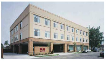
Because of seismic conditions in the Pacific Northwest, the Emerson House Residential Care Facility in Portland, Ore., was constructed with a precast modified moment-frame system. The system expedited construction on the tight urban site during rainy winter months. Photo: Bob Boll Photography
